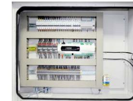
Easy accessible electrical cabinet is integrated in the unit. Only well known and reliable components from ABB, Schneider electric and PLC from Carel (Italy) or EVCO (Italy) or SIEMENS (Germany) are utilized.
